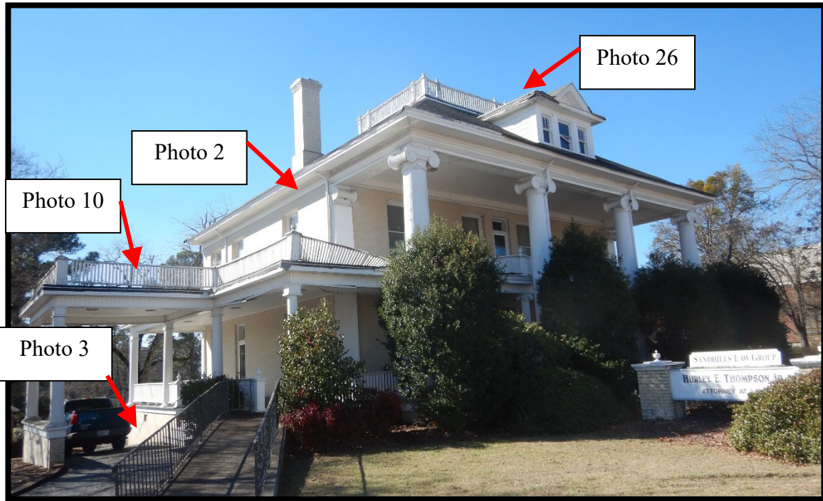
Photo #1 - This is the front of 208 Monro St.
