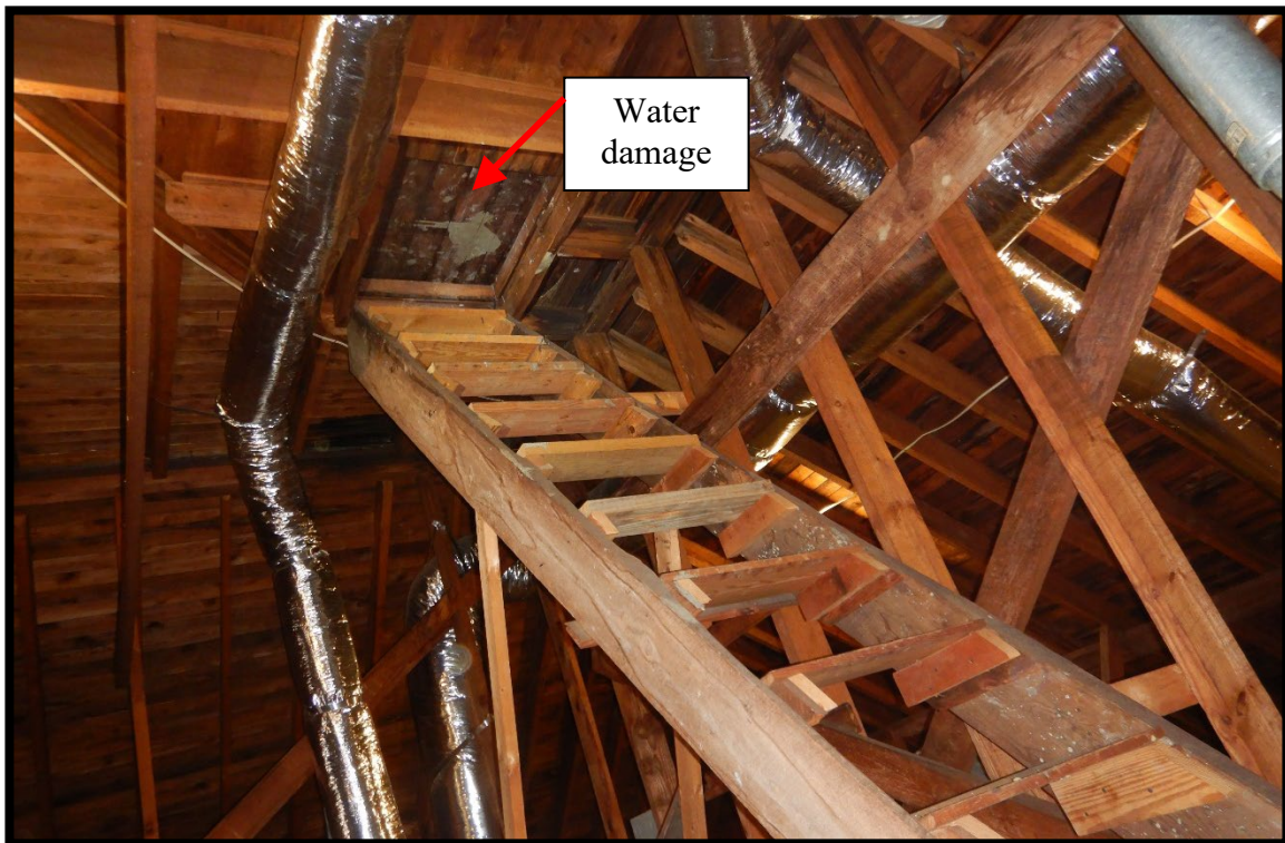
Photo #32 – Stairs to the top flat roof. The access will need rebuilding. The stairs were not safe.
