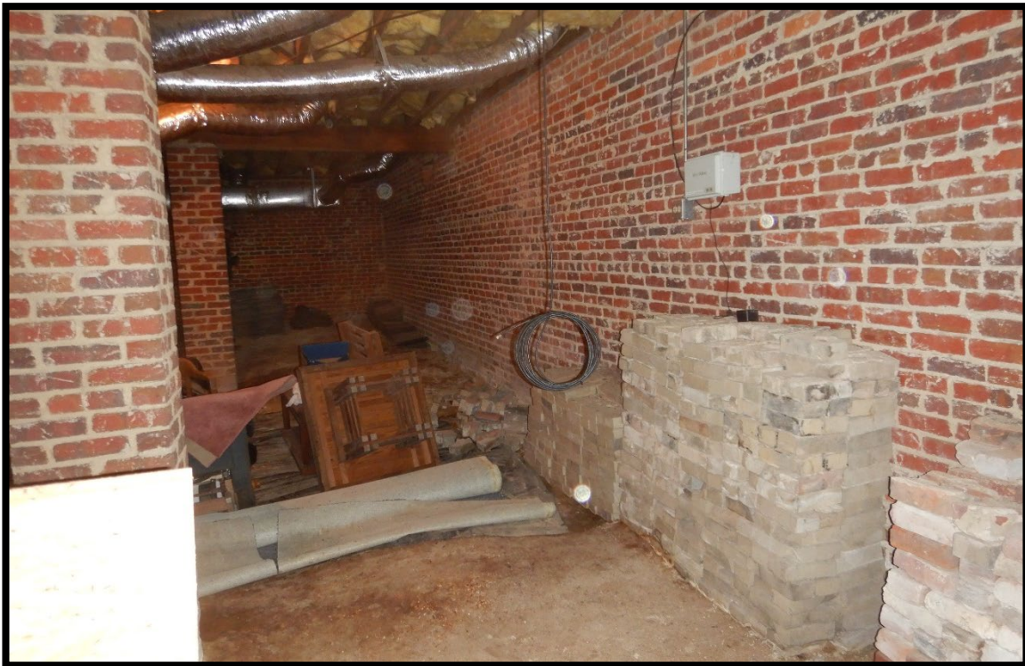
Photo #16 - This is the foundation wall along the right side.
