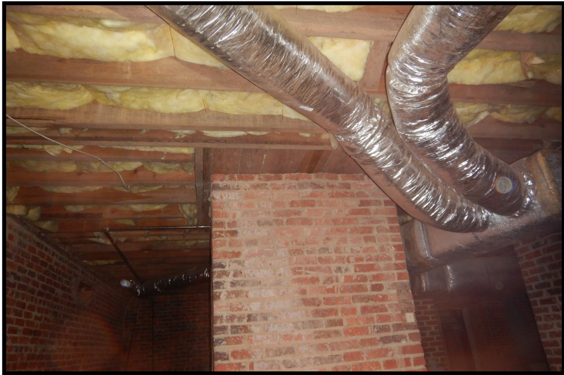
Photo #17 - This is a photo of the chimney foundation
