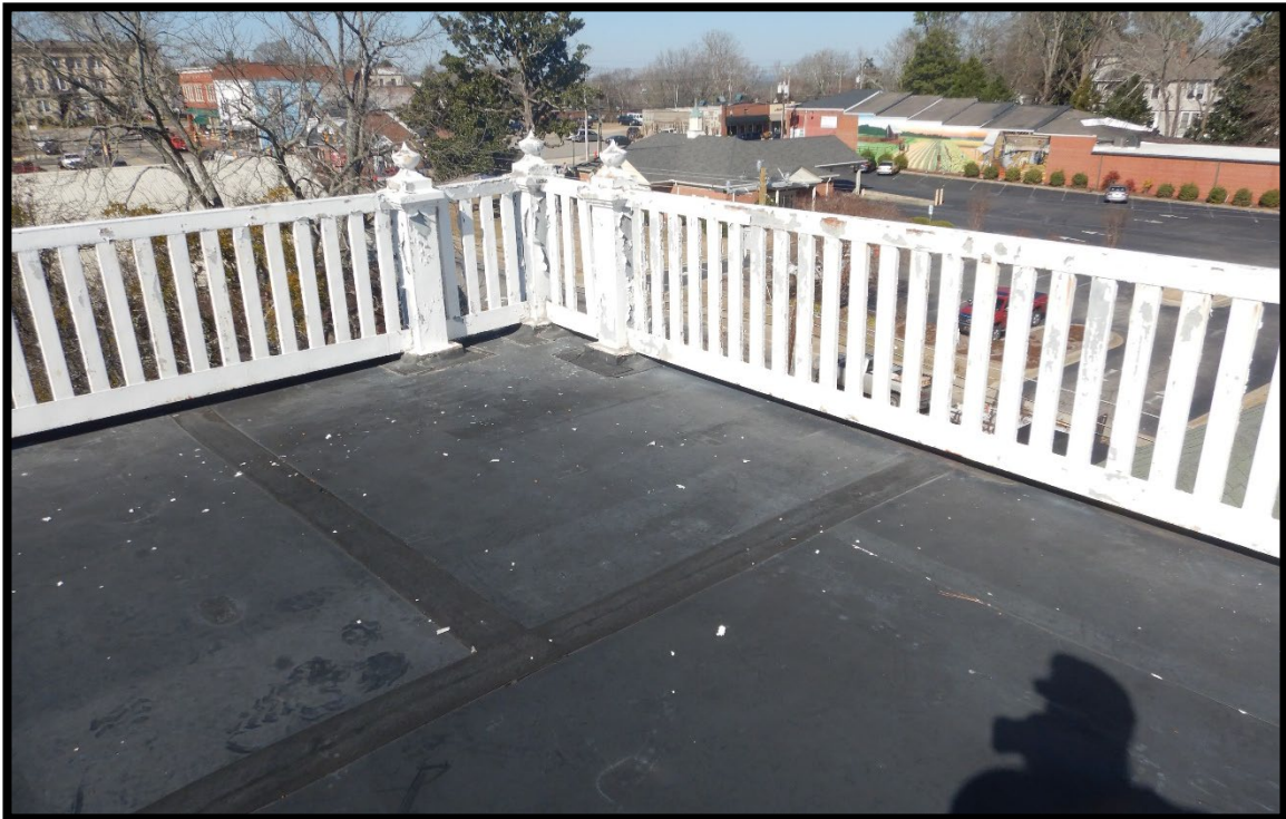
Photo #24 - Top roof railing.
